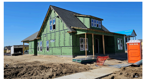
Construction Update: February 2025
