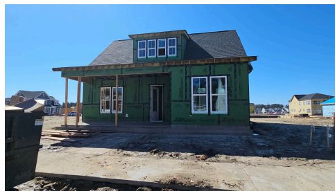
Construction Update: February 2025
