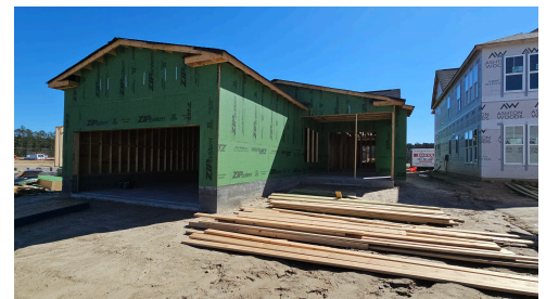
Construction Update: February 2025
