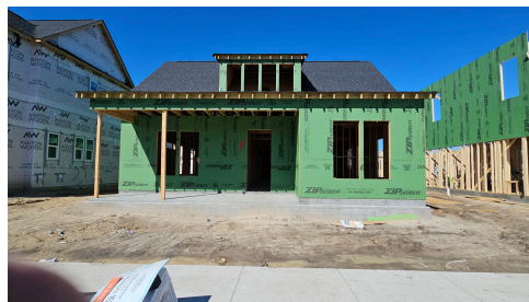
Construction Update: February 2025
