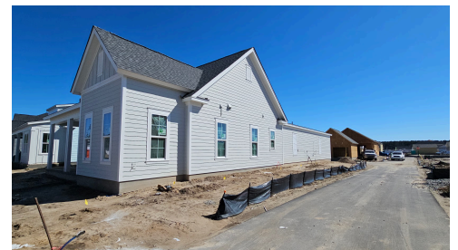
Construction Update: February 2025
