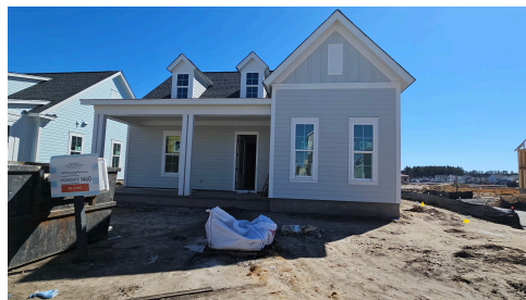
Construction Update: February 2025
