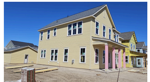
Construction Update: February 2025
