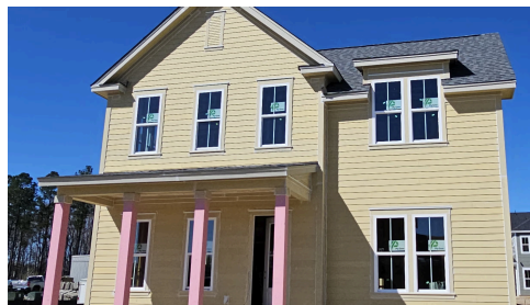
Construction Update: February 2025
