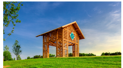
Wendell Falls Entrance
