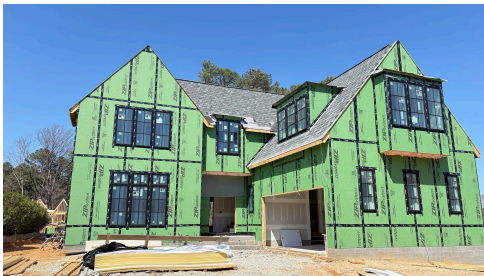
Construction Update: March 2025
