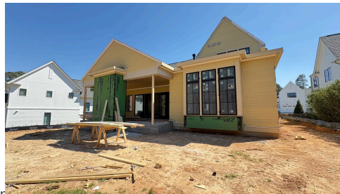
Construction Update: March 2025
