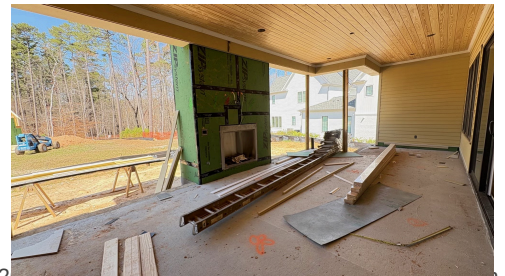
Construction Update: March 2025
