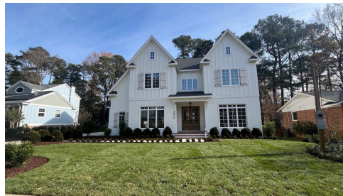
Construction Update: Dec 2024
