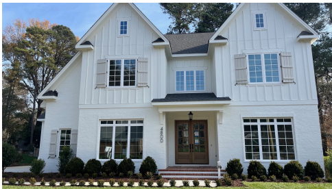
Construction Update: Dec 2024
