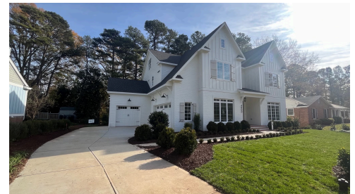
Construction Update: Dec 2024
