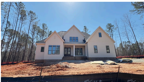
Construction Update: March 2025
