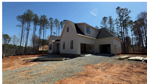
Construction Update: March 2025
