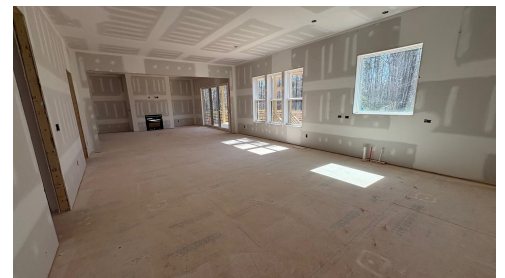
Construction Update: March 2025
