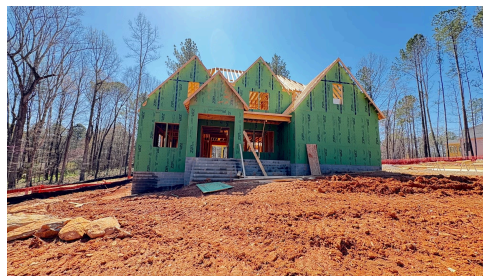
Construction Update: March 2025
