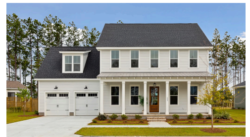
Example of completed home
