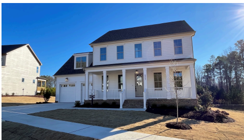
Construction Update: January 2025
