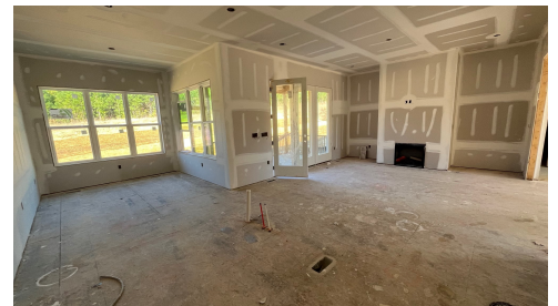
Construction Update: October 2024
