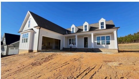
Construction Update: January 2025
