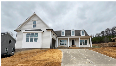
Construction Update: March 2025
