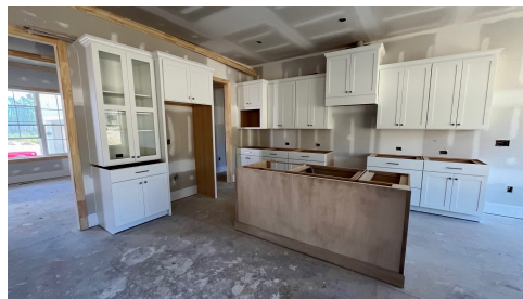
Construction Update: January 2025
