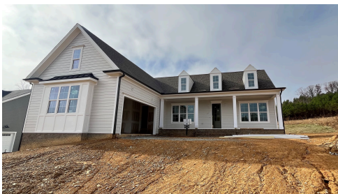
Construction Update: December 2024
