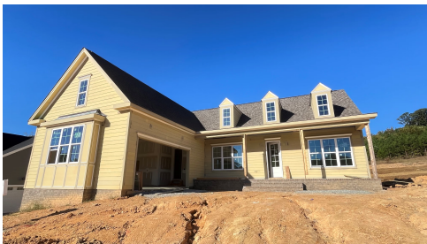
Construction Update: October 2024
