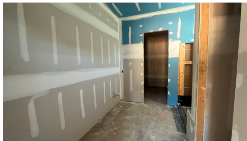
Construction Update: October 2024
