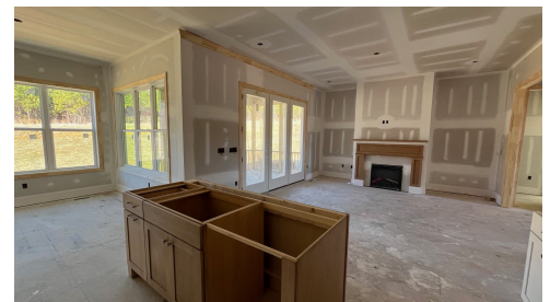
Construction Update: January 2025
