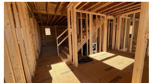
Construction Update: January 2025
