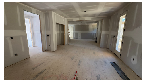
Construction Update: March 2025
