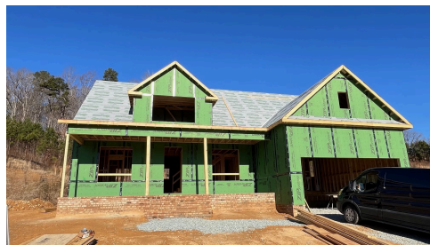
Construction Update: January 2025
