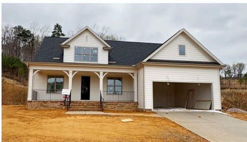
Construction Update: March 2025
