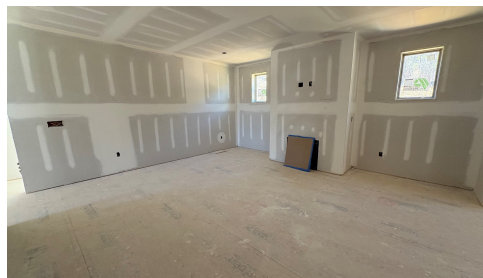
Construction Update: March 2025
