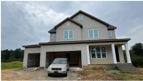
Construction Update: August 2024
