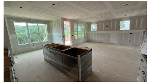
Construction Update: August 2024
