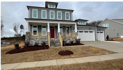
Construction Update: December 2024
