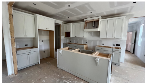
Construction Update: August 2024
