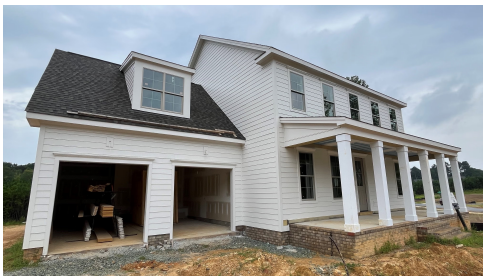
Construction Update: August 2024
