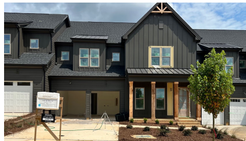
Construction Update: September 2024
