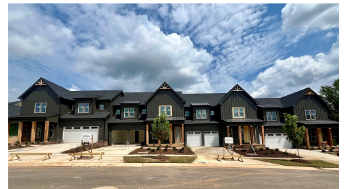
Construction Update: September 2024
