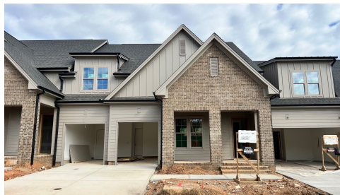
Construction Update: Nov 2024
