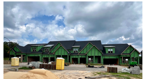
Construction Update: August 2024
