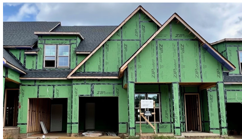
Construction Update: August 2024
