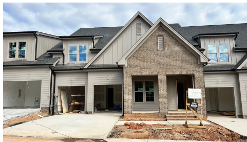
Construction Update: Nov 2024
