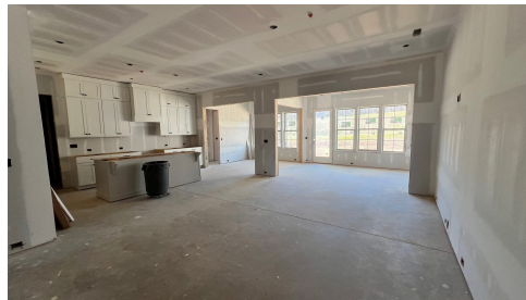
Construction Update: March 2025
