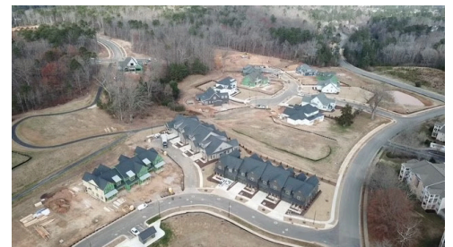
Community Construction Update: Dec 2024
