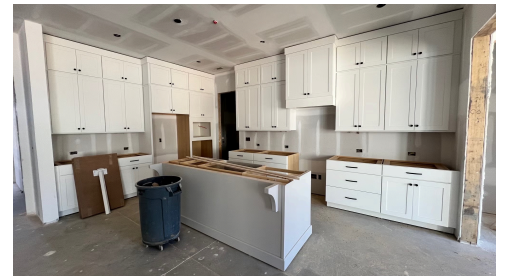
Construction Update: March 2025
