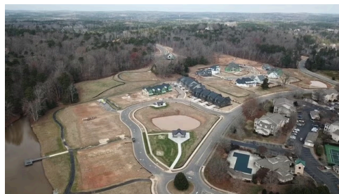
Community Construction Update: Dec 2024
