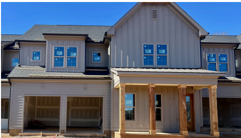
Construction Update: March 2025
