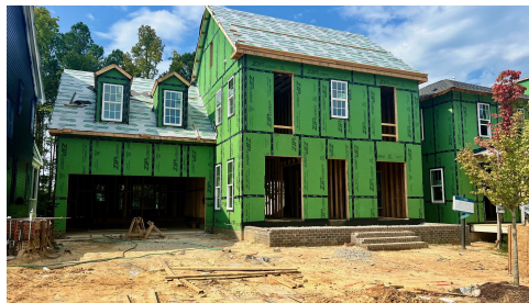
Construction Update: August 2024
