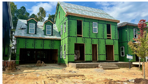
Construction Update: August 2024
