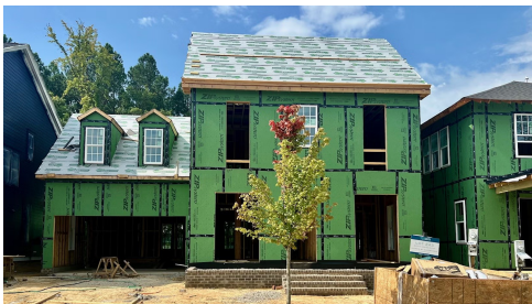
Construction Update: August 2024
