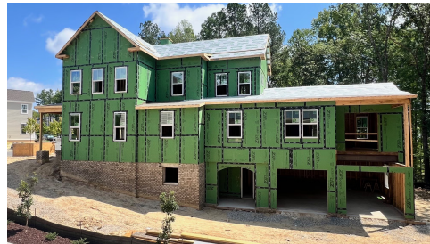
Construction Update: August 2024
