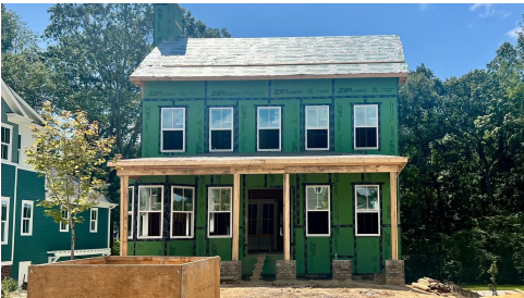
Construction Update: August 2024
