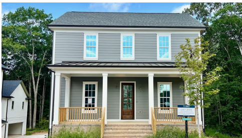
Construction Update: August 2024
