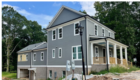
Construction Update: August 2024
