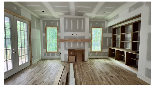
Construction Update: August 2024
